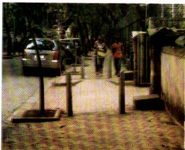
Fig. 16 Footpaths with Side Ramps at Property Entrance in Mumbai
