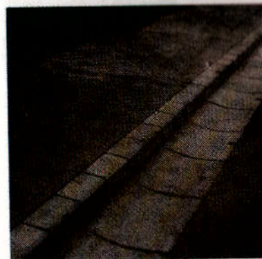
Fig. 27 Kerb Stone Block with Saucer Drain
