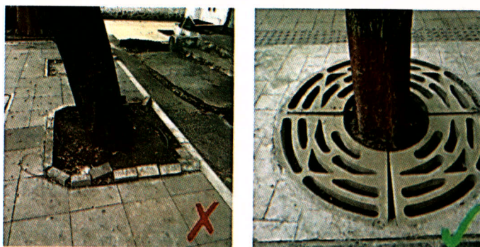
Fig. 54 Tree Grating Detail
